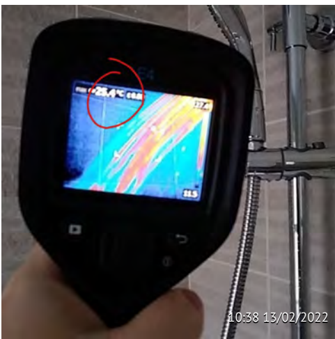
74 Shower trade Plumber Low water temp
