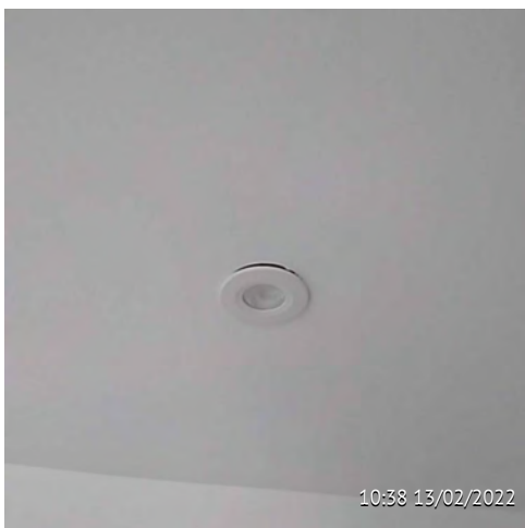
80 Bathroom trade Decorator Make good decorative finish to ceiling
